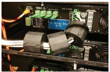
Figure 2. Ferrite chokes help decouple cross-coupled switching noise away from amplifier outputs.
