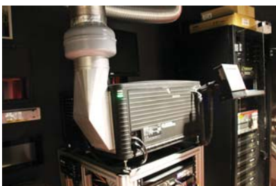
The projection booth equipped with Christie Digital Projector, GDC Server, GDC IMB, Dolby Digital Processor and QSC Audio System
