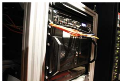
The projection booth equipped with Christie Digital Projector, GDC Server, GDC IMB, Dolby Digital Processor and QSC Audio System
